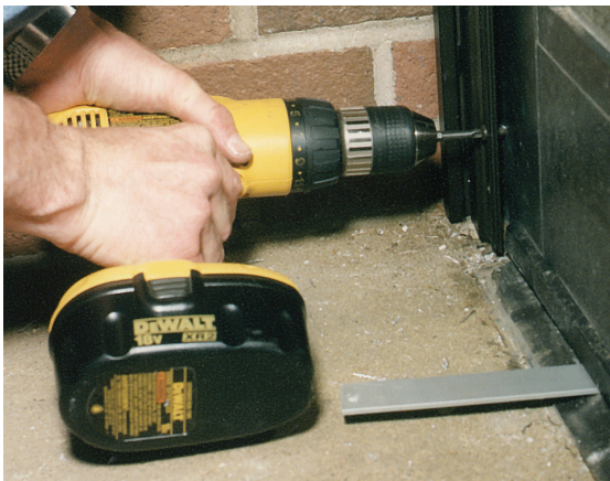
▲ Installing the bottom locator screw in the door leaf. Note the shim supporting the door, assuring proper threshold clearance.
