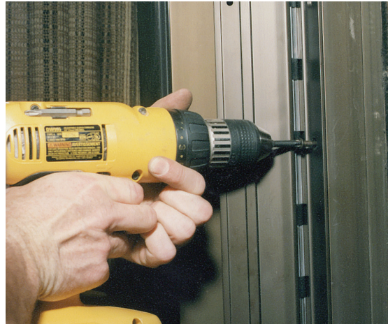
▲ Installing screw in frame leaf. Hinge is in open position, showing hinge bearings.
