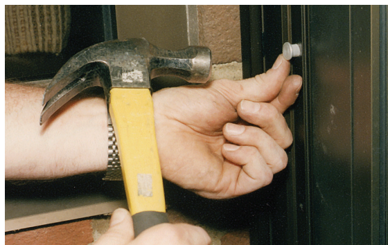
▲ Tapping in the barrel half of a through-bolt to secure the door leaf to the outside of the door.
