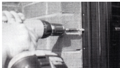
10] Driving self-drilling screws.
