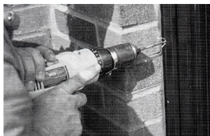
9] Drilling pilot holes.
