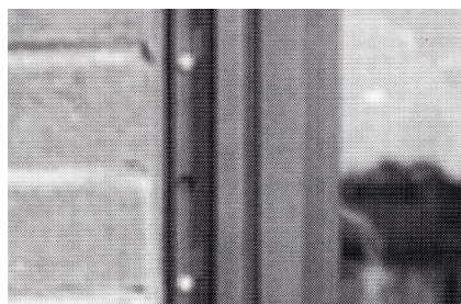
11] Showing pan head screws.
