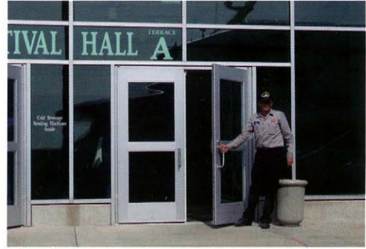
Don Johnson, carpenter foreman at Navy Pier, stands in front of newly-installed Special-Lite doors.
