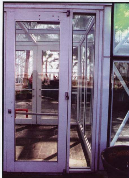
These photos show how strong winds have destroyed internal door reinforcements for pivots. MPEA carpenters were creative and used hardwood blocking inside storefront doors to reattach pivots as a temporary fix. This was the first door that Special-Lite replaced.
