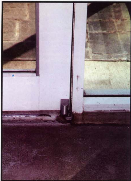
These photos show how strong winds have destroyed internal door reinforcements for pivots. MPEA carpenters were creative and used hardwood blocking inside storefront doors to reattach pivots as a temporary fix. This was the first door that Special-Lite replaced.
