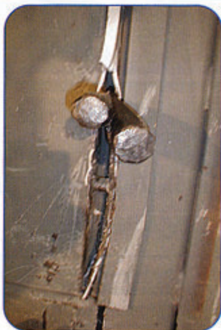
4. A 9 x 2 1/2-in. wood-splitting wedge was used.
