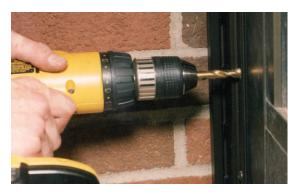
▲ Drilling fastener hole through door leaf hole into face of door.
