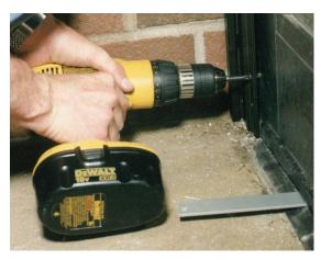
▲ Installing the bottom locator screw in the door leaf. Note the shim supporting the door, assuring proper threshold clearance.
