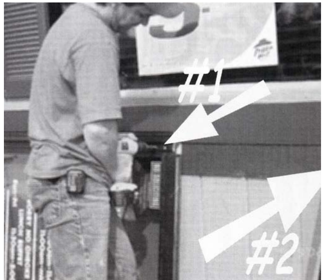
5] Securing hinge with self-drilling screws.
