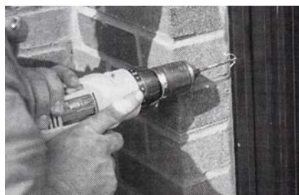
9] Drilling pilot holes.
